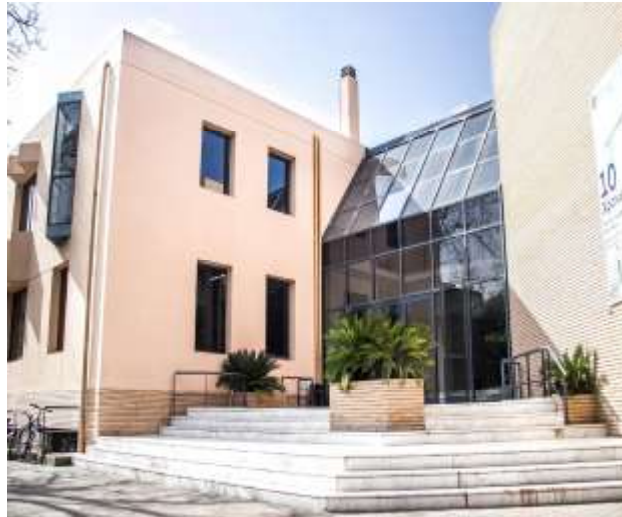
The building where the Department of Geography is located
